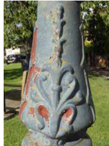
Figure 84: Street lamp requiring repainting, Little Green
