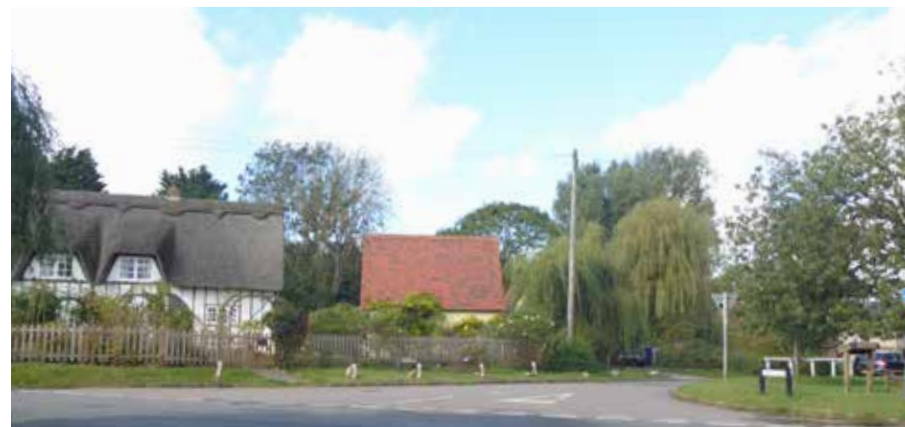
Figure 89: Poorly proportioned modern outbuildings detract from the appreciation of their host dwellings
