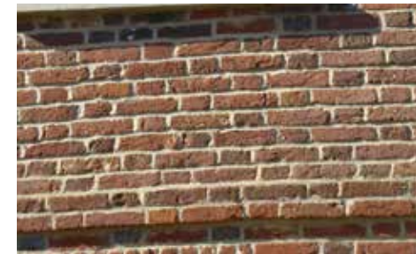
Figure 33: example of Flemish bond brickwork, common within the Character Area
