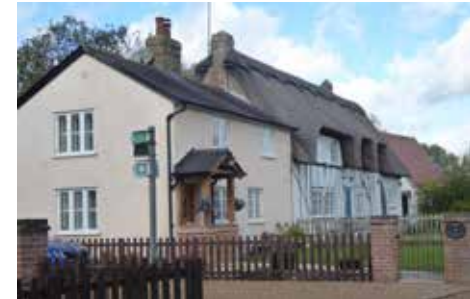
Figure 37: Roof coverings within the Character Area are varied yet predominantly traditional
