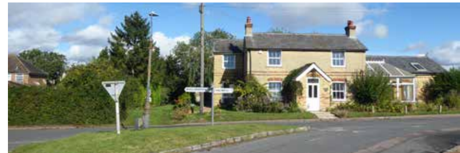
Figure 13: Holwell Road, proposed to be added to the Conservation Area
