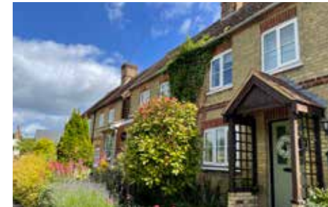
Figure 72: example of where uPVC windows mimic traditional window types
