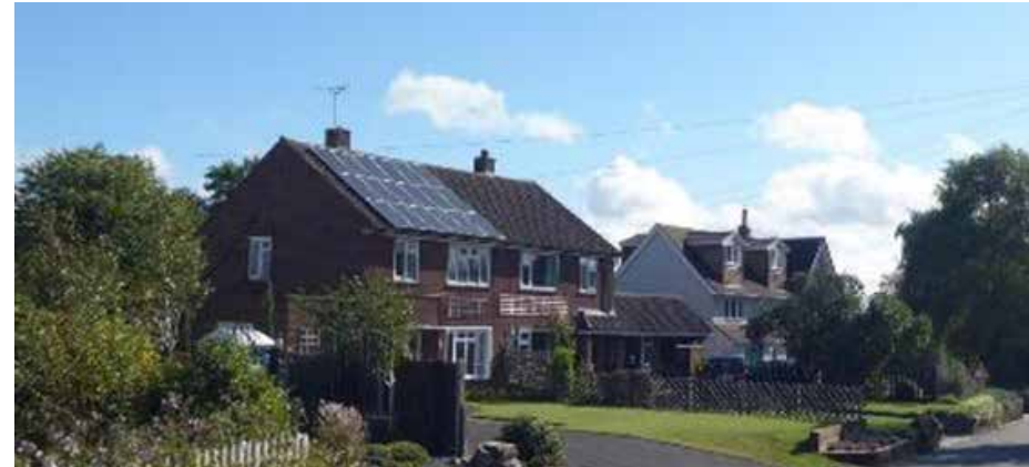
Figure 12: Properties on Hitchin Road, suggested for removal from the removed from the Conservation Area
