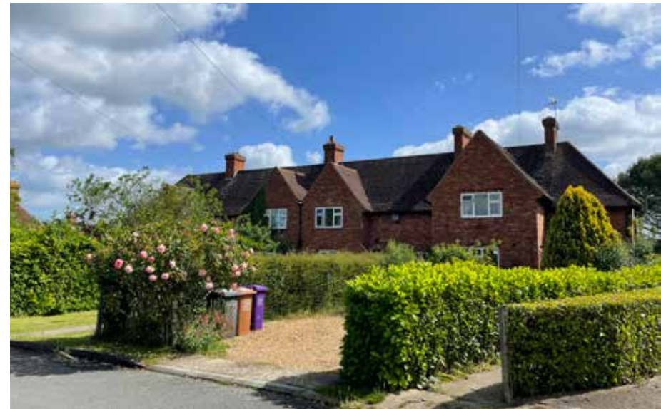
Figure 14: Houses on Davis Close, which are proposed to be added to the Conservation Area
