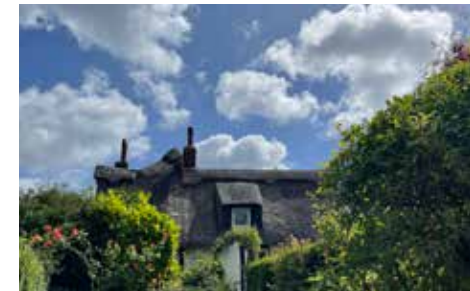
Figure 62: 17 High Street, largely concealed from the road due to its elevated position
