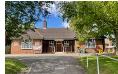
Figure 60: The Village Hall, High Street
