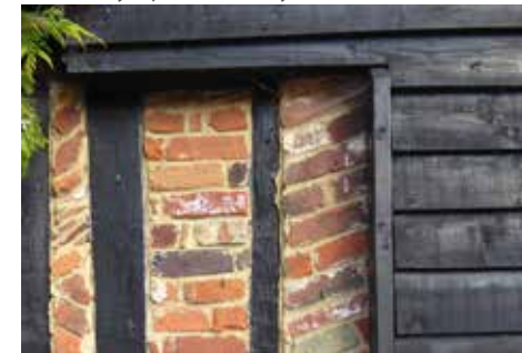
Figure 38: An example of exposed timber framing and brick nogging, found throughout the Character Area
