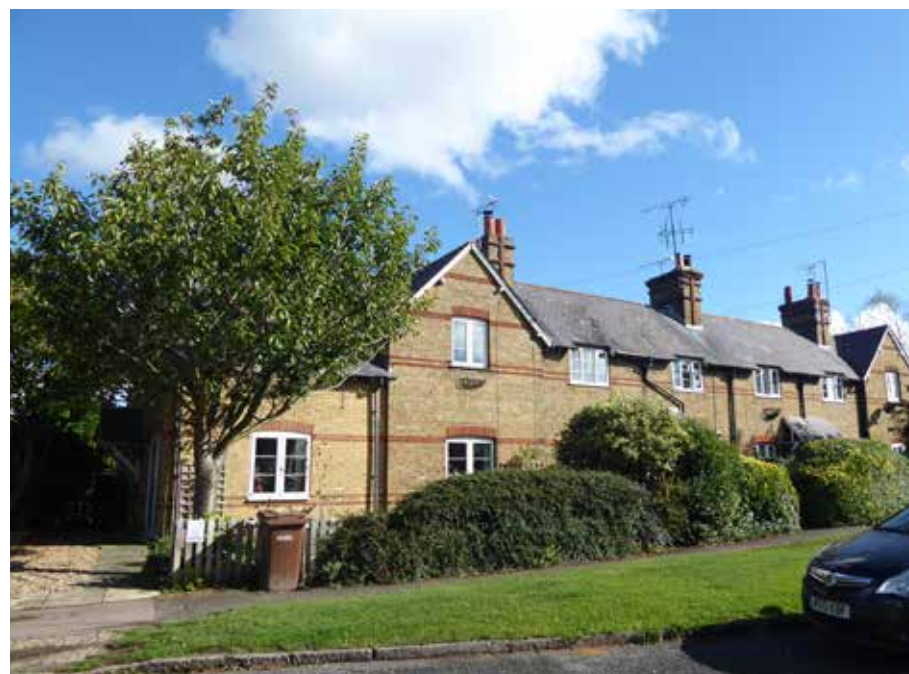
Figure 18: Nineteenth century cottages on the High Street, built in local Arlesey white brick with decorative red brick banding
