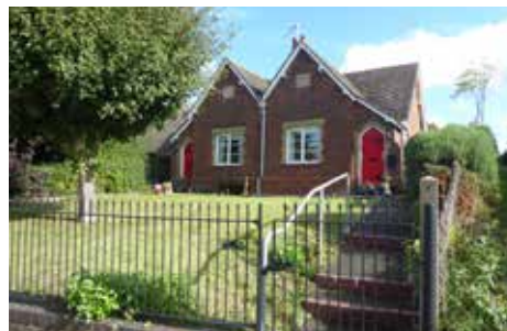
Figure 66: 19 and 21 High Street
