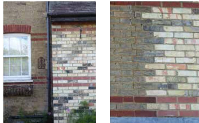
Figure 88: Poorly matched, bright modern brick, can contrast poorly next to original buildings if not well considered
